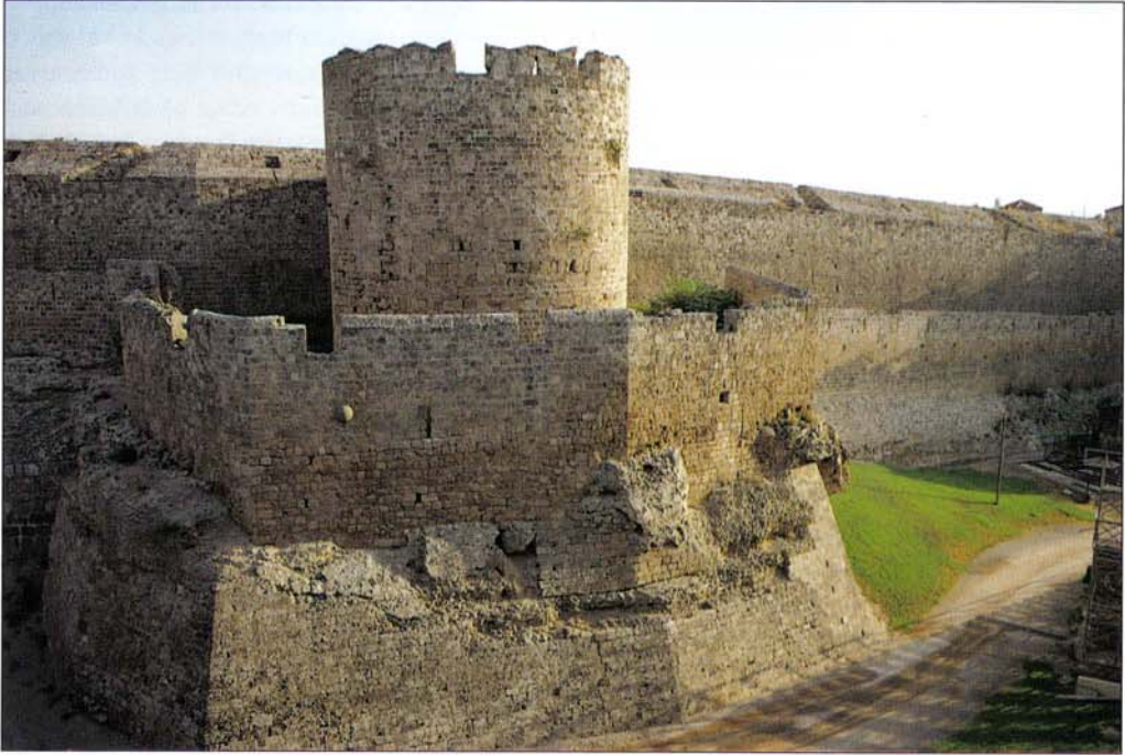
A round tower in the land walls of Rhodes.
